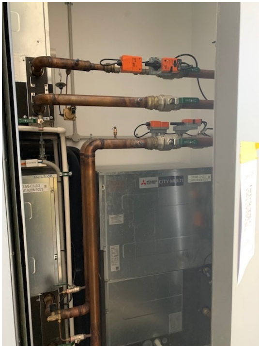
PQHY system installed within unventilated service cupboards, as it does not require ventilation.
