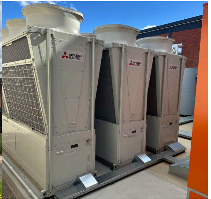
Mitsubishi Electric EACV-M1500YCL E-series Modular Chillers in place for the Mildura Arts Centre chilled water plant replacement project.
