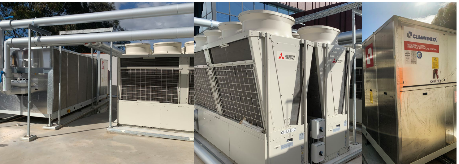
ERACS2 System & E-Series units providing hot water supply.
