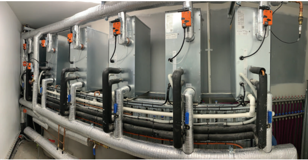
CITY MULTI PWFY HEX (Heat Exchanger) units.
